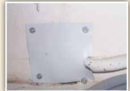
Power supply hole sealed with metal flashing.*
