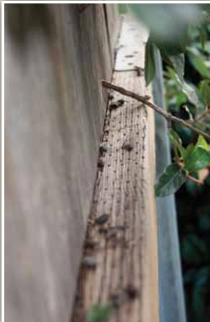
Droppings on fenceline.
