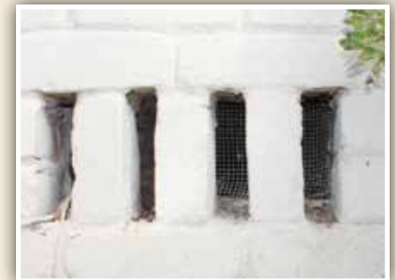
Check for loose mesh in foundation vents.
