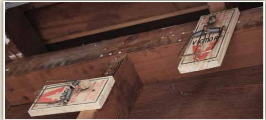
Proper trap placement on beams and rafters. Note rub marks on beams indicating rat trails.
