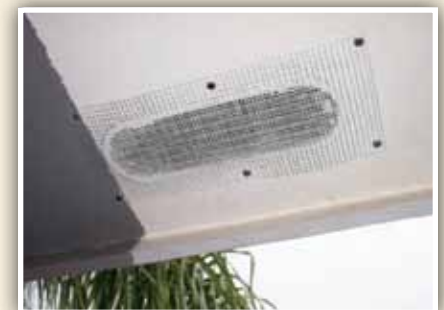
Soffit vent hole sealed with screen.*
